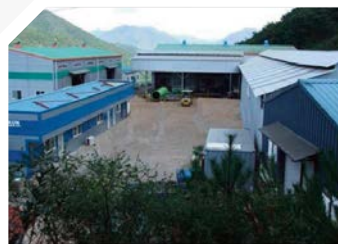
TSA Coating Factory
